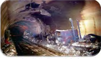
Ruins of the Mont-Blanc tunnel fire (1999) Fire duration: 53h; Fatalities: 39 (including a firefighter and a security guard).
